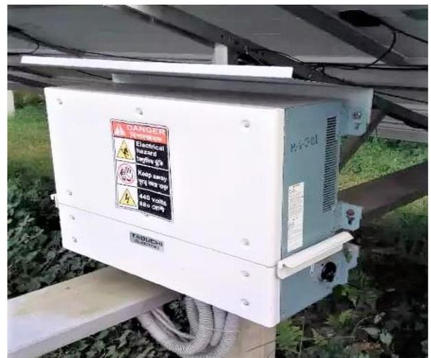
Photo: Installed Inverter below the installed solar PV panels.
