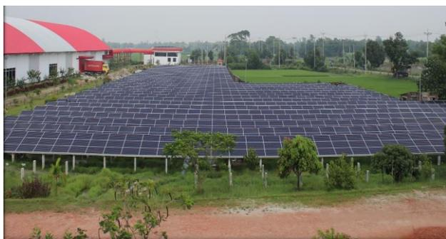
**Photo:** Installation ground mounted solar PV panels (890 kWp) at FESIL factory premise at Madhabpur, Habiganj district.
