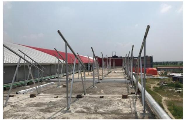
**Photo:** Mounting structure installation works of solar PV panels at the factory rooftop of FESIL at Madhabpur, Habiganj district
