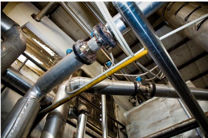
Steam Flowmeter setup for steam Monitoring
