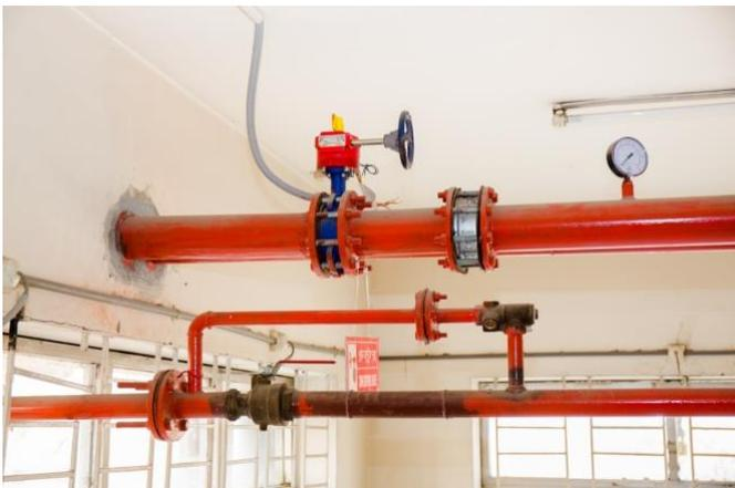
*Zone Control Valves to control Sprinklers waterflow or malfunctions at the factory floor of Divine Textile Ltd*
