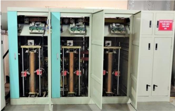
**Photo:** AVR (Automatic Voltage Regulator) voltage regulator and stabilizer in the factory in case of voltage fluctuations in the grid, which also supports the smooth operation of the grid tied inverters.
