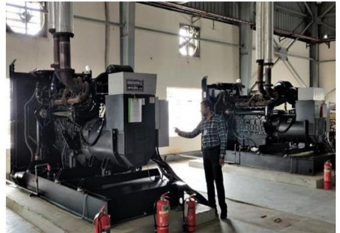
Photo: 2 X 750 kVA diesel generators, runs during the load shedding hours, Electricity from solar PV systems reduces the load of these generators during load shedding hours
