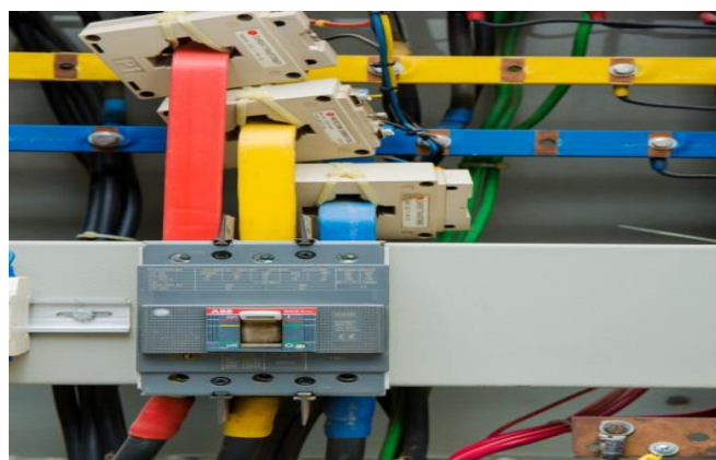
MCCB (Molded Case Circuit Breaker) with CT for MDB
