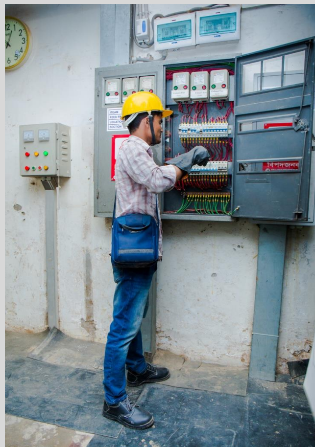
Electrical works on circuit breaker with safety
